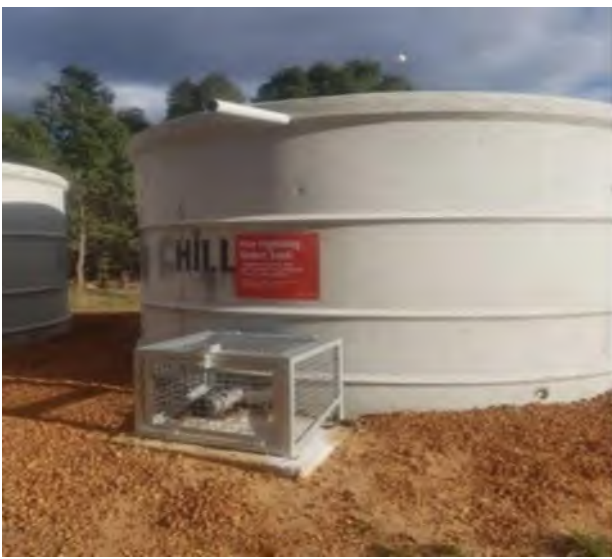
Strategic 47,000 Litre Concrete Tank & Protected Fittings
