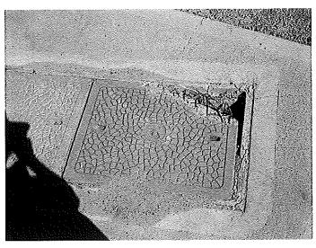
Service/manhole access covers in concrete paths are generally uneven. This photo was of an extreme case of damage.
