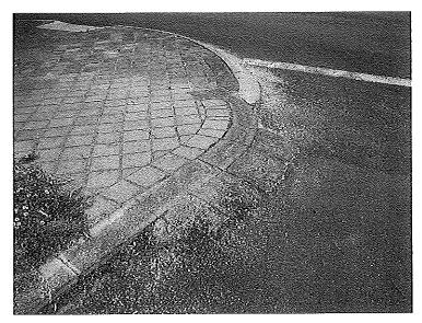
On and off ramps at road intersections are uneven and can cause wheelchairs to tip. The intersection at the corner of Adam and Warren St is of particular concern.
