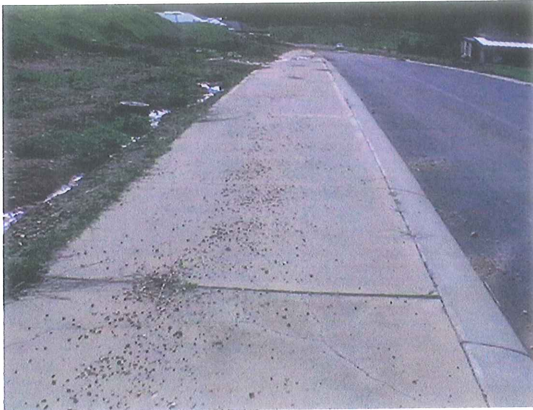
Figure 9. Erosion Adjacent to Footpath in Hitchcock Drive
