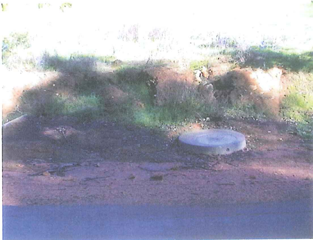
Figure 8. Erosion Adjacent to Brockman Hwy
