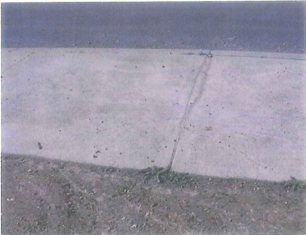
Figure 6. Footpath Damage Severity 2
