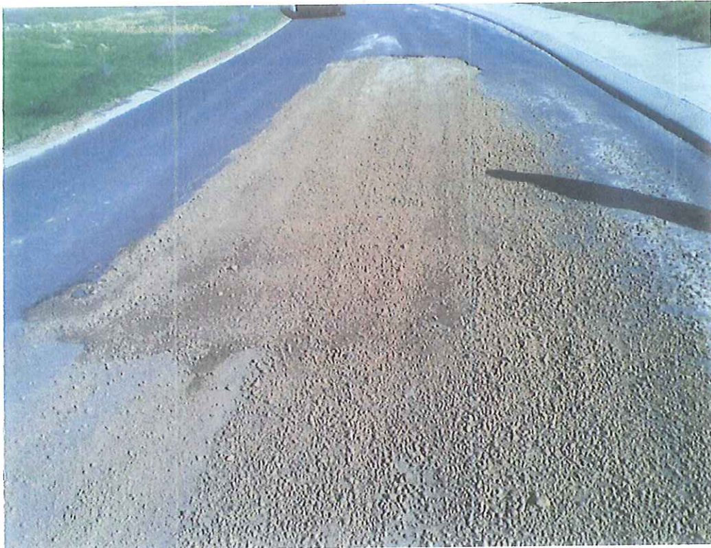
Figure 4. Pavement Damage Severity 3
