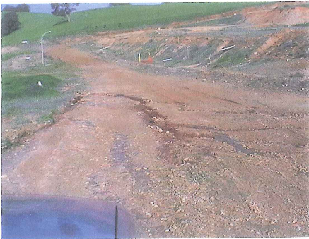
Figure 2. Pavement Damage opposite POS
