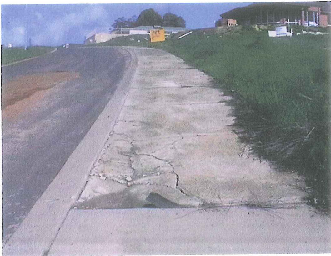
Figure 4. Pavement Damage Severity 3
