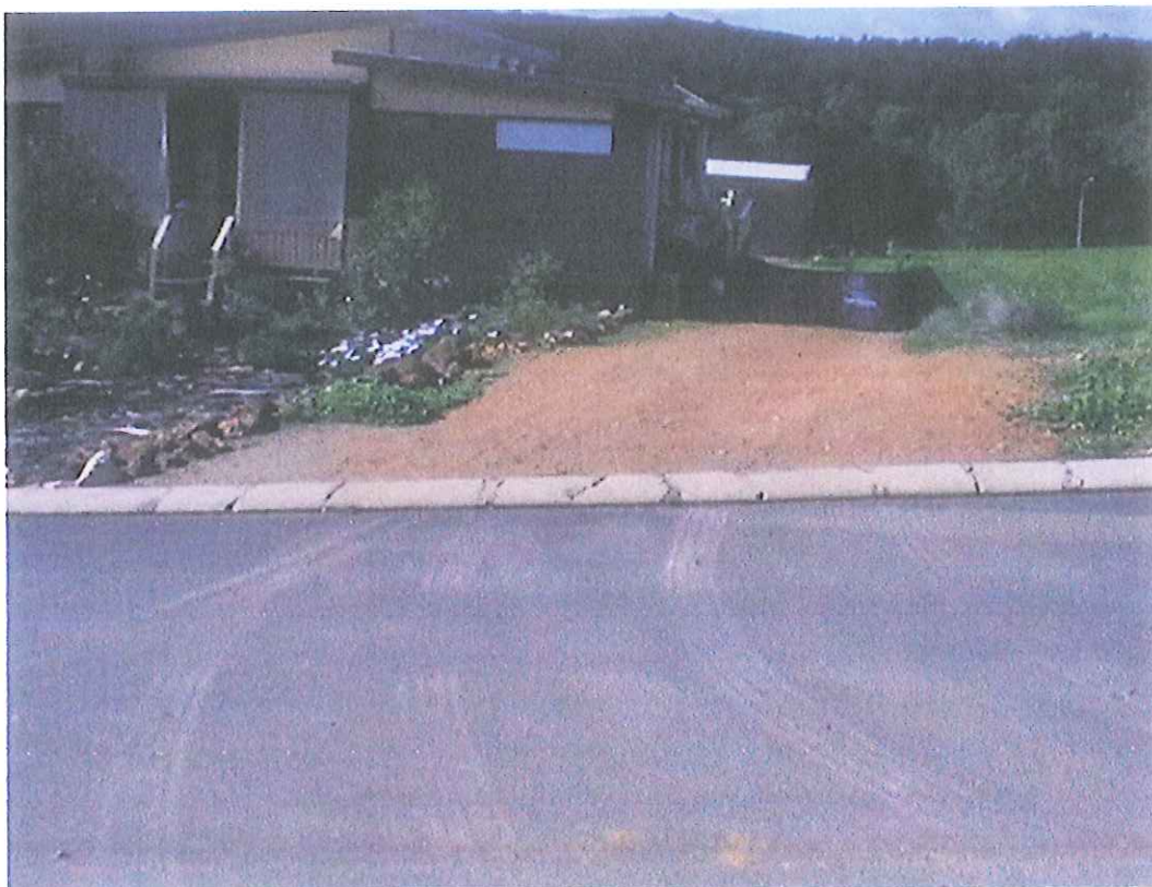
Figure 7. Kerb Damage Severity 3
